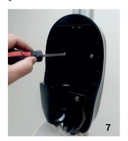
Open the automatic dispenser with the push-in key. Remove gel bottle. Align the fixing holes with the bracket and tighten the two small screws.
